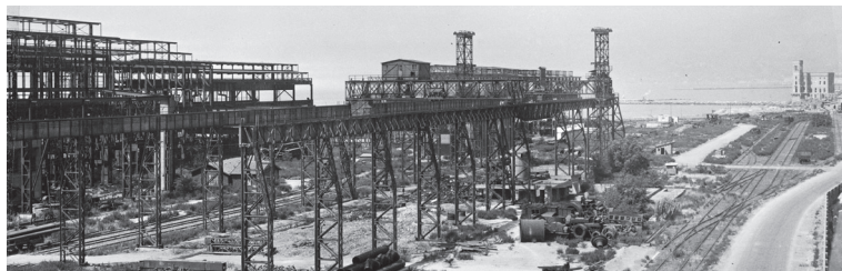
20 October 1950: infilling occurring within sight of Castello Raggio (Archivio Storico Fondazione Ansaldo)
